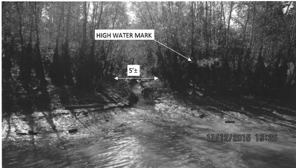
Fig. 5: Photo taken in 2015 at Element 3 from the Atchafalaya River during low water showing the high water mark on willow trees that have germinated within the channel bed. The cleared water bottom width is approximately 5'.
